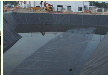
RCC Tank Lining
